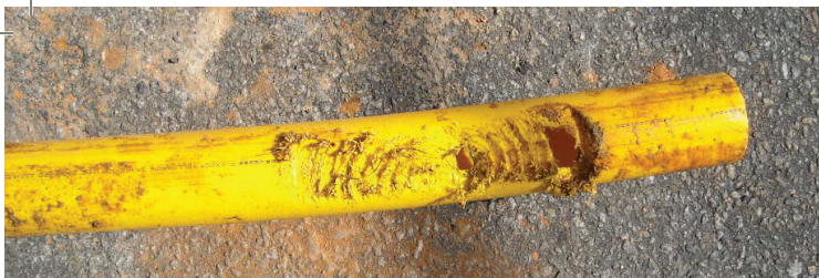
Natural gas piping damaged during cleaning operations
