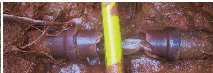
A sewer line penetrated by natural gas piping
